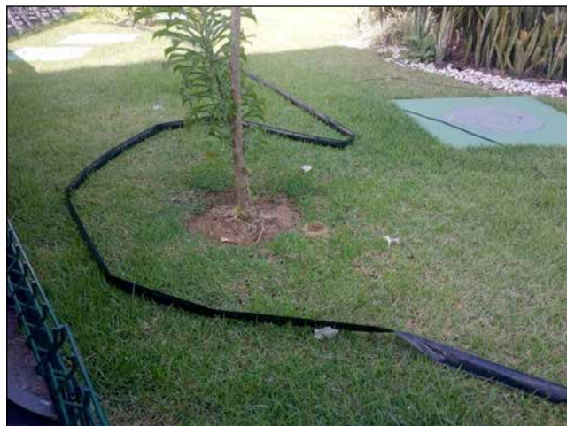
Figure 9. Black irrigation hose installed in the garden bed, manually perforated for water release.
