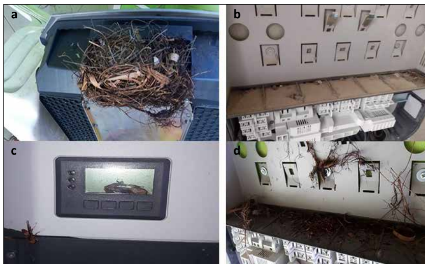
(a) interruption by a bird's nest; (b) interruption by a frog; (c) interruption by building material; (d) interruption by dry leaves.
