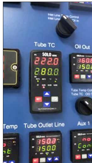
Figure 3. Programmable Logic Controller (PLC).
